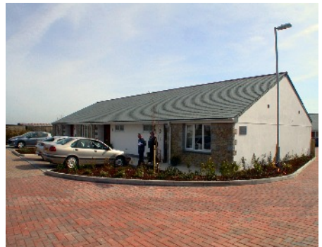
Part of the £1 million development at Mills Gardens
